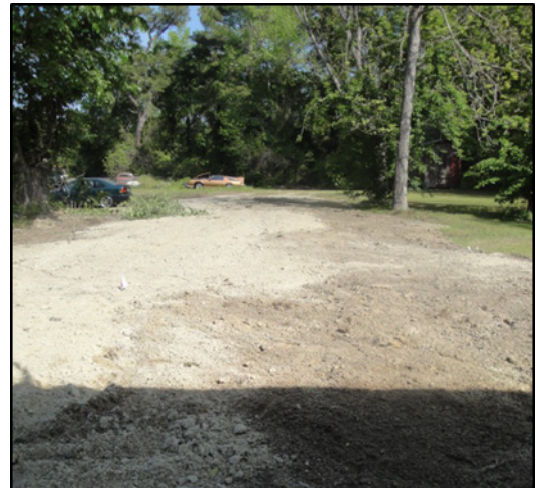
Before (above) and after (below) pictures showing washing machine line in yard (also discharged under the house) and after new ultrashallow system was installed to treat all household wastewater (site will revegetate).
