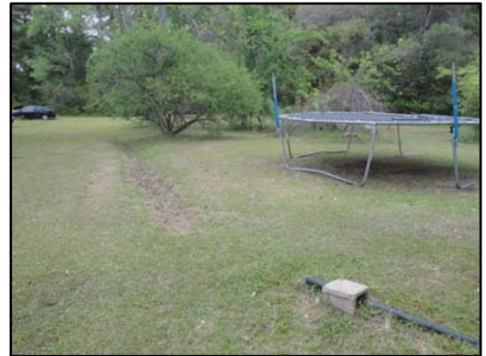
Before (above) and after (below) pictures showing washing machine line in yard (also discharged under the house) and after new ultrashallow system was installed to treat all household wastewater (site will revegetate).
