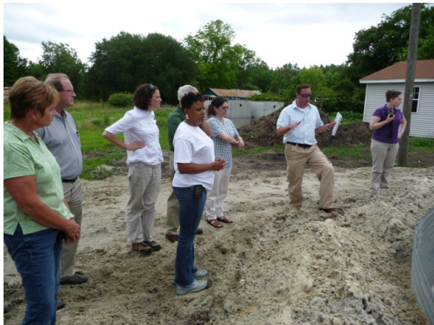
First Year Site Visit held September 2010. Committee looks at septic installation site. Project partners site visit attendees included: EPA, SC DHEC, Dept. of Natural Resources, Charleston Soil & Water Conservation District, Charleston Resource Conservation and Development, and SC Coastal Conservation League.
